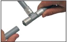
2. Insert the pipe into the fitting. Ensure you push the pipe all the way (15mm) into the shoulder of the fitting.
