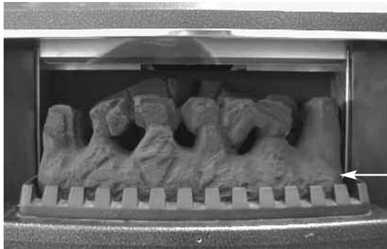
Fuelbed front section fits behind the front casting as shown
